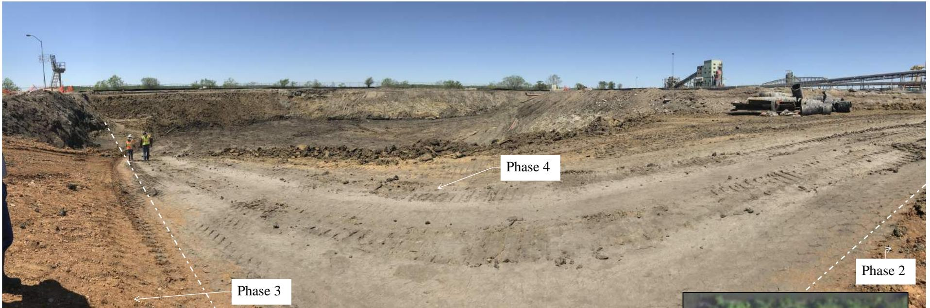
Photo was taken on May 8, 2020, at a centrally-located point from within the Impoundment, looking north/ north-east, at the completion of CCR removal. Backfill of the Phase 3 area can be seen to the west of the viewpoint. Clay was observed at the base of the unit. Survey information for this phase was taken on May 8, 2020.
