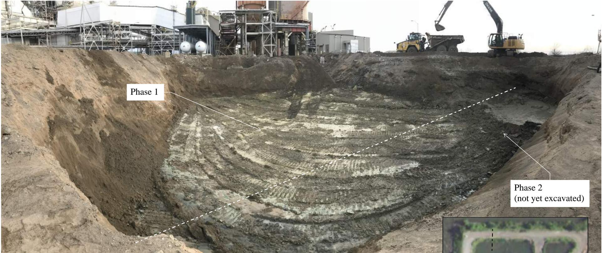
Photo was taken on February 11, 2020, from the east side of the Impoundment looking south-west, during a pause in CCR removal operations. Clay is observed at the base of the unit. Survey information for this phase was taken on February 20 and February 28, 2020, after which the backfill of the Phase 1 area began.
