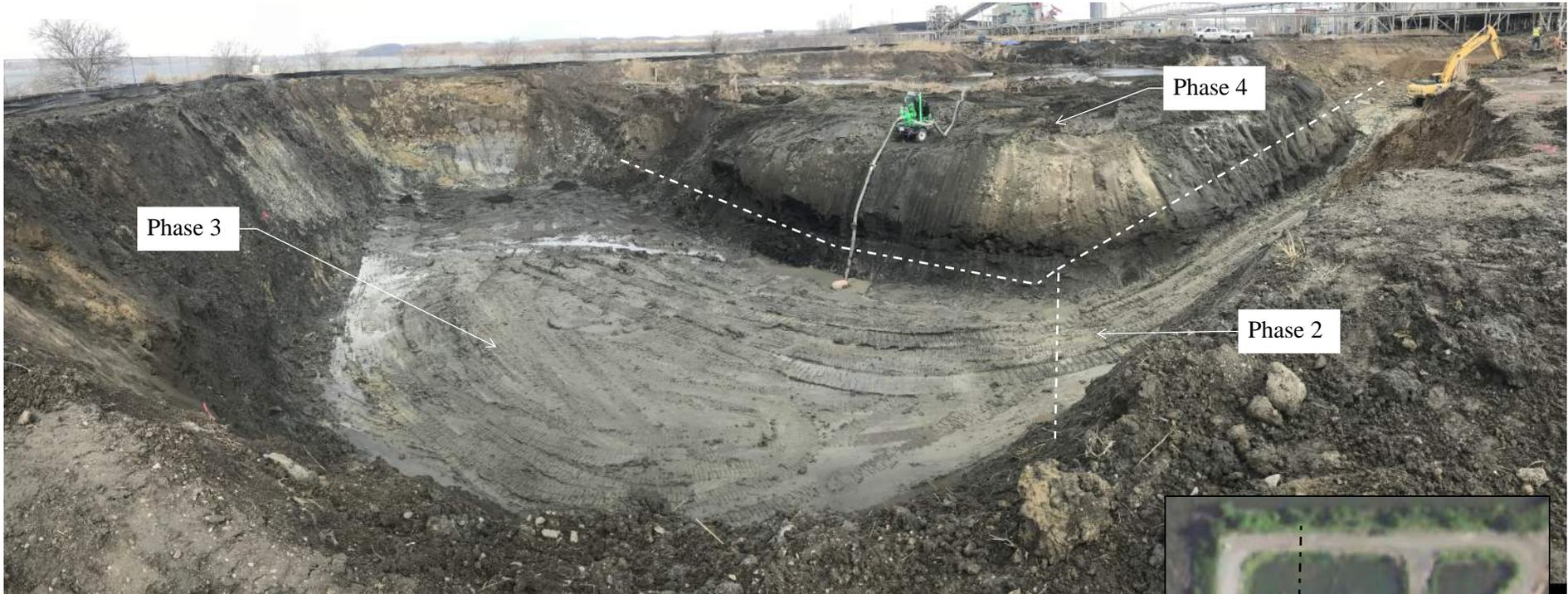
Photo was taken on March 12, 2020, from a point on the west berm of the Impoundment, looking north/north-east, during a pause in CCR removal as well as Phase 1 backfill operations. Clay was observed at the base of the unit. Survey information for this phase was taken on March 13, 2020, at which point backfill operations of the Phase 3 area commenced so as to improve the physical/ hydraulic barrier separating the Impoundment and La Cygne Lake.
