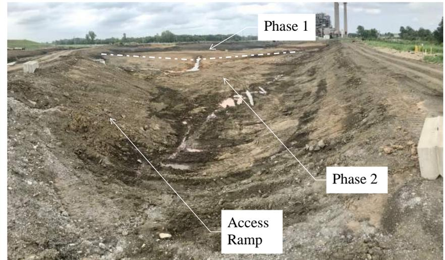
Photos were taken on June 29, 2020, from the west side of the Ash Impoundment looking east and south and north and east, respectively, following the completion of CCR removal operations of the South Ash Impoundment. Clay is observed at the base of the unit. Survey information for this phase was taken on July 2, 2020.
