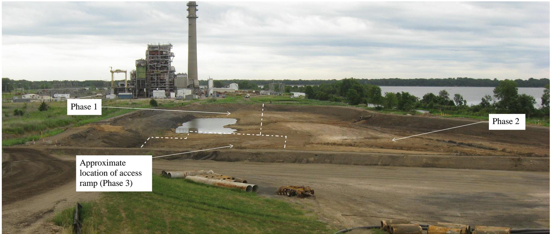
Photo was taken on July 9, 2020, from the west side of the North and South Ash Impoundments looking east, following the completion of removal of the access ramp (Phase 3). Clay was observed at the base of the unit in all locations. Survey information for this phase was taken on July 14, 2020.
