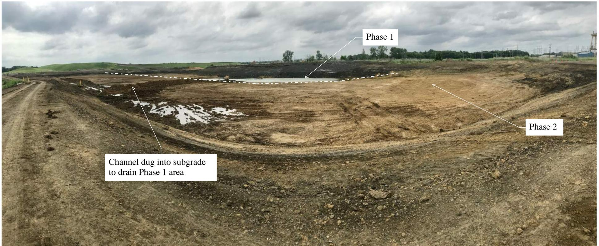
Photo was taken on June 29, 2020, from the south-east corner of the South Ash Impoundment looking west to north, following the completion of CCR removal operations of the South Ash Impoundment. Clay is observed at the base of the unit. Survey information for this phase was taken on July 2, 2020.
