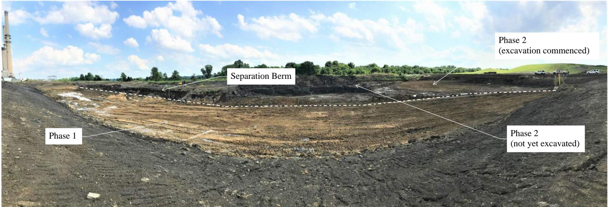
Photo was taken on June 9, 2020, from the west side of the Ash Impoundment looking east and south, following the completion of CCR removal operations of the North Ash Impoundment. Clay is observed at the base of the unit and a portion of the separation berm is observed on the eastern end. Survey information for this phase was taken on June 12, 2020.
